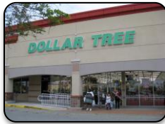
Dollar Tree Commercial Painting - Interior, Various Locations South Florida
