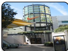
Nike Town Commercial Painting - Interior, 3 Story 25,000sf
