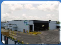
Waste Services Of Florida, Inc Franklin Rodriguez, Manager Industrial Painting
