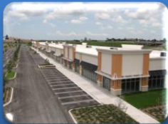
Homestead Pavillion Shopping Center HRC Construction New Construction - Exterior Painting TexCote Cool Wall
