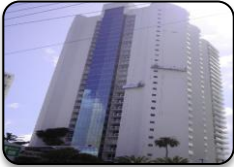
Oceania Tower I Commercial Painting - 32 Story High-Rise Building, Exterior Waterproofing
