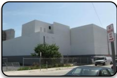
Warehouse Building Commercial Painting - Exterior
