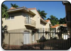
Grove Walk Condominium Commercial Painting - Town House Condo Exterior Painting
