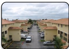
Tamarind Grove Condominium Commercial Painting - 6 Buildings Exterior Painting & Sealcoating
