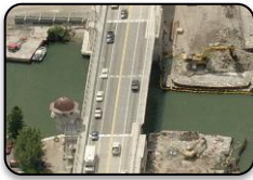
12 Ave Bascule Bridge Commercial Painting - Interior
