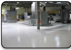
Propulsion Technology Commercial Painting - Industrial Epoxy Floors
