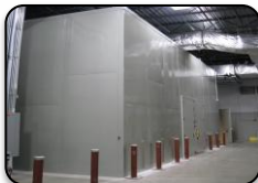
Eckel Industries, Inc Florida Heat Pump Sound Room Industrial Painting
