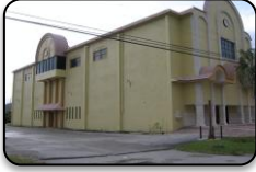
Hialeah Church Commercial Painting - Exterior
