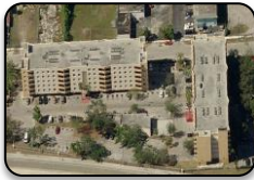
Edison Terrace I & II Commercial Painting & Concrete Restoration- Exterior
