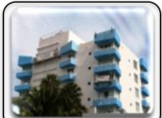
Ocean Place Condominium Commercial Painting - 8 Story Mid-Rise Building, Exterior Painting
