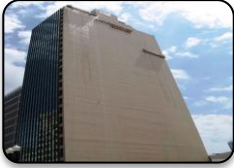
Court House Tower Commercial Painting - 28 Story High-Rise Building, Exterior Waterproofing
