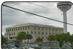
Miccosukee Tribe Health Care Building Commercial Painting- Exterior
