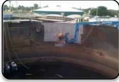
Cooper City Surge Tank WWTP Industrial WWTP Painting
