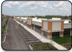
Homestead Pavillion Shopping Center New Construction - Exterior Painting TexCote Cool Wall
