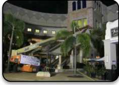
Aventura Mall Commercial Painting- Exterior Painting
