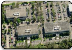
Parkside Buildings I, II & III Graham Companies Commercial Painting - Exterior- Multiple Properties
